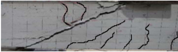
Fig. 15. Modes of failure for ferrocement beams (Shear compression failure).
